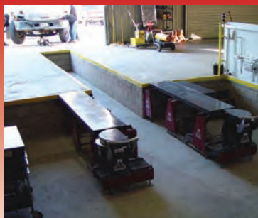
Typical Two Section T-Style Pit
